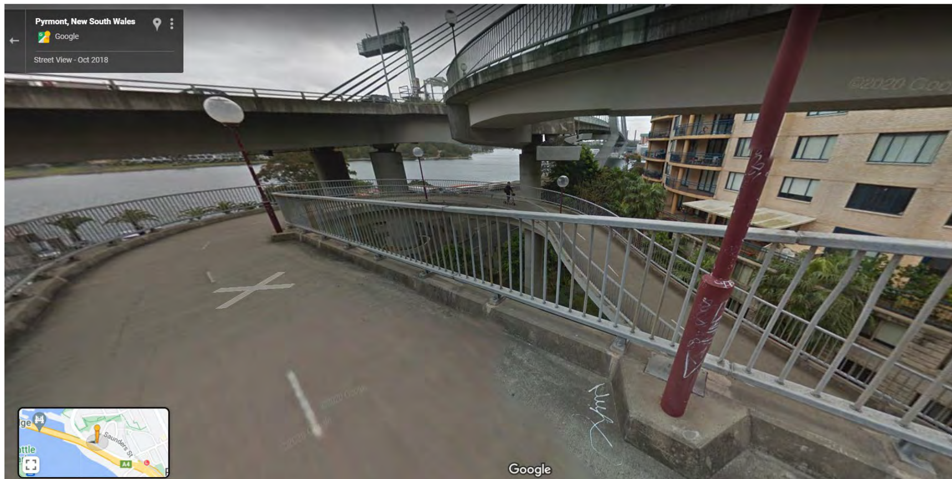
Anzac Bridge Cycle Ramp – Inside Structure radius – 6.0m approx. Width varies, 3.60m av. Gradient varies, 5-8 % approx. Length 180m approx.
