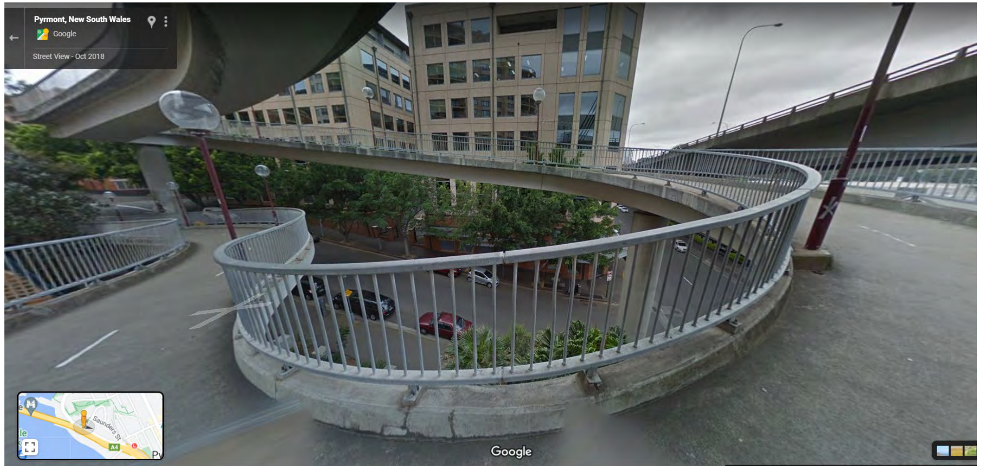
Anzac Bridge Cycle Ramp – Inside Structure radius – 6.0m approx. Width varies, 3.60m av. Gradient varies, 5-8 % approx. Length 180m approx.
