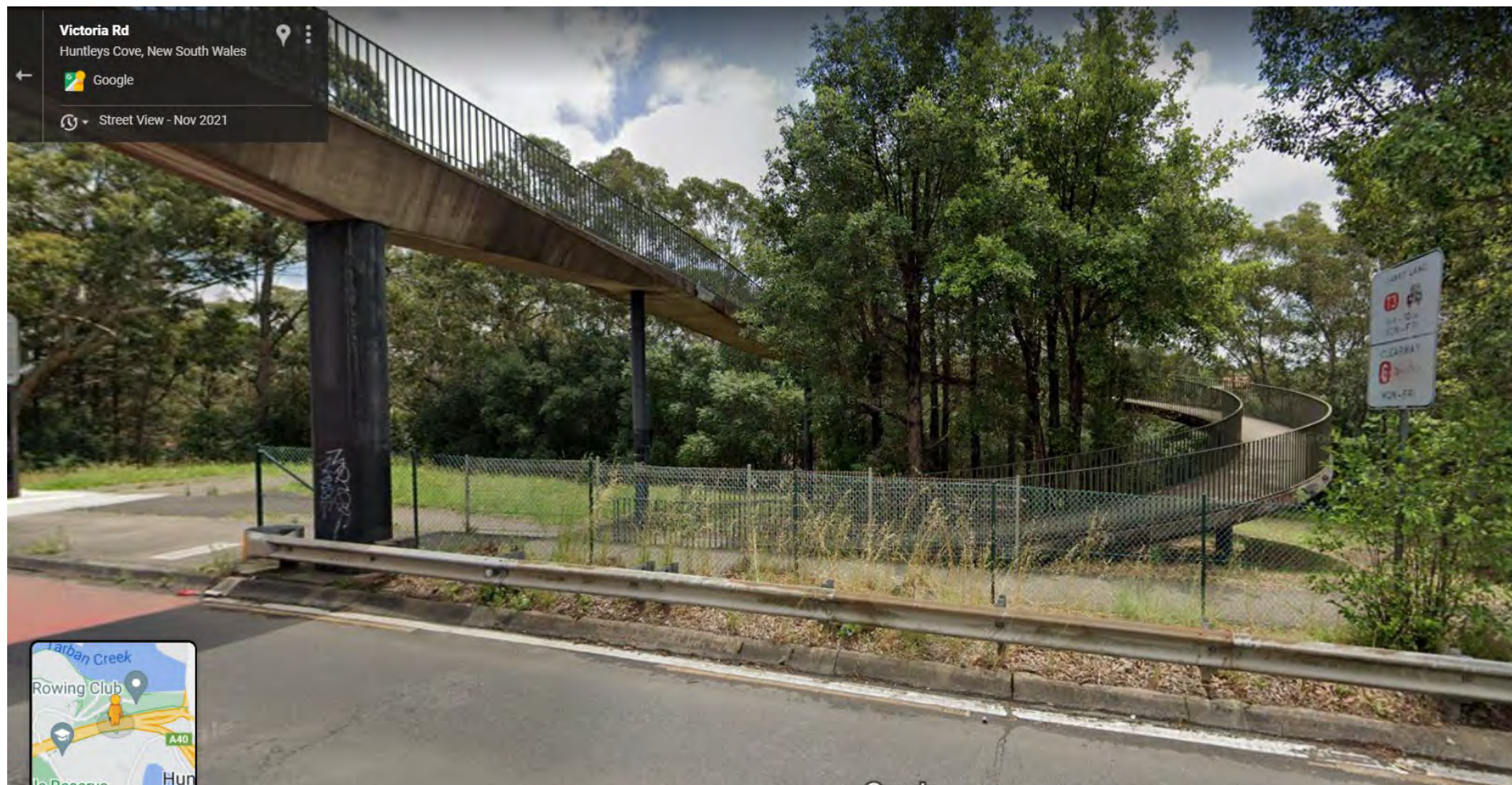
Victoria Road Huntleys Point – inside structure radius – 7.0m approx., width 2.0m approx
