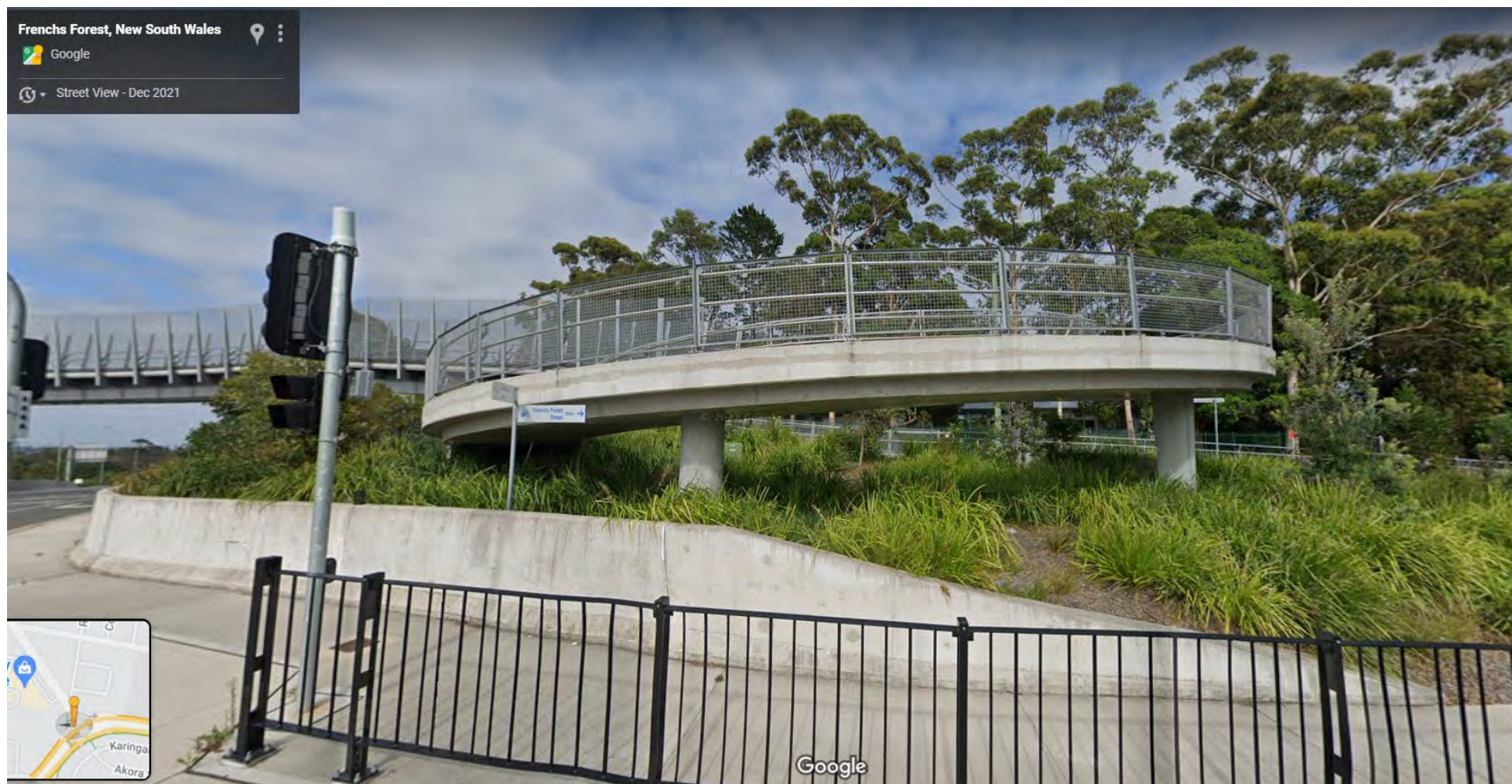
Forest Way Frenchs Forest – Compound Curve Ellipse (inside structure radii - 6m & 8.5m approx.) Width 3.0m approx.
