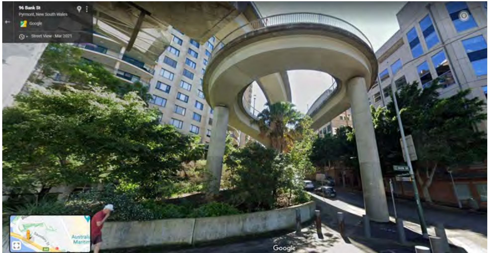
Anzac Bridge Cycle Ramp – Inside Structure radius – 6.0m approx. Width varies, 3.60m av. Gradient varies, 5-8 % approx. Length 180m approx.
